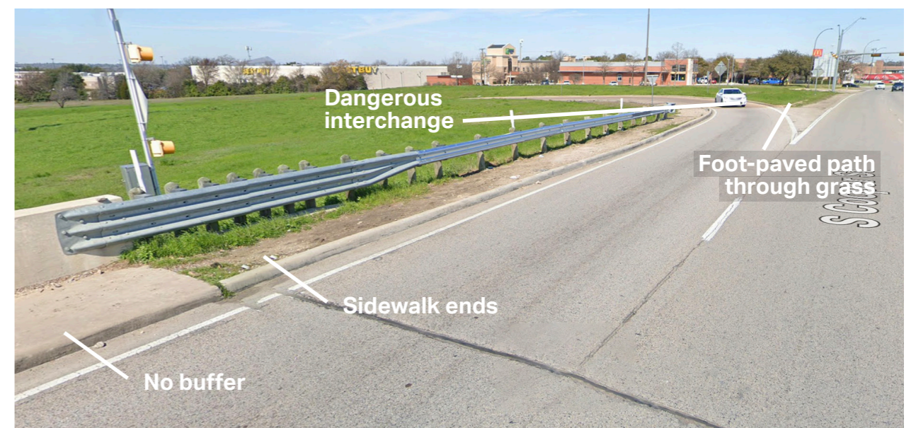
Figure 78: IH-20 Existing Conditions Source: Google Earth
