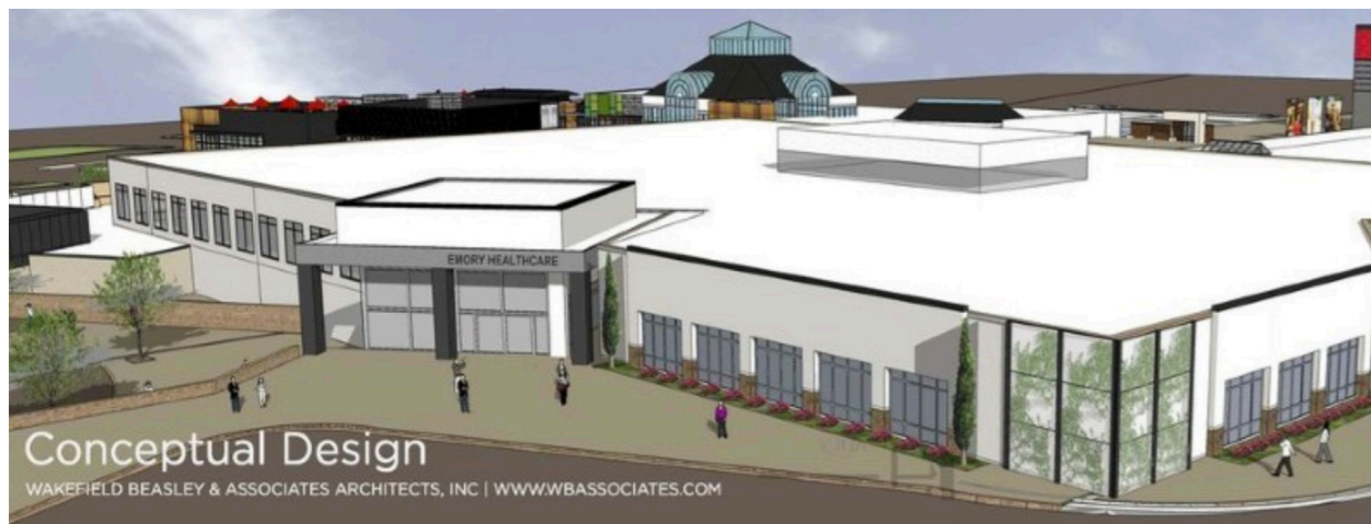
Figure A3-8: Conceptual Design for Emory Healthcare in North Lake Mall Source: Atlanta Real Estate Forum
