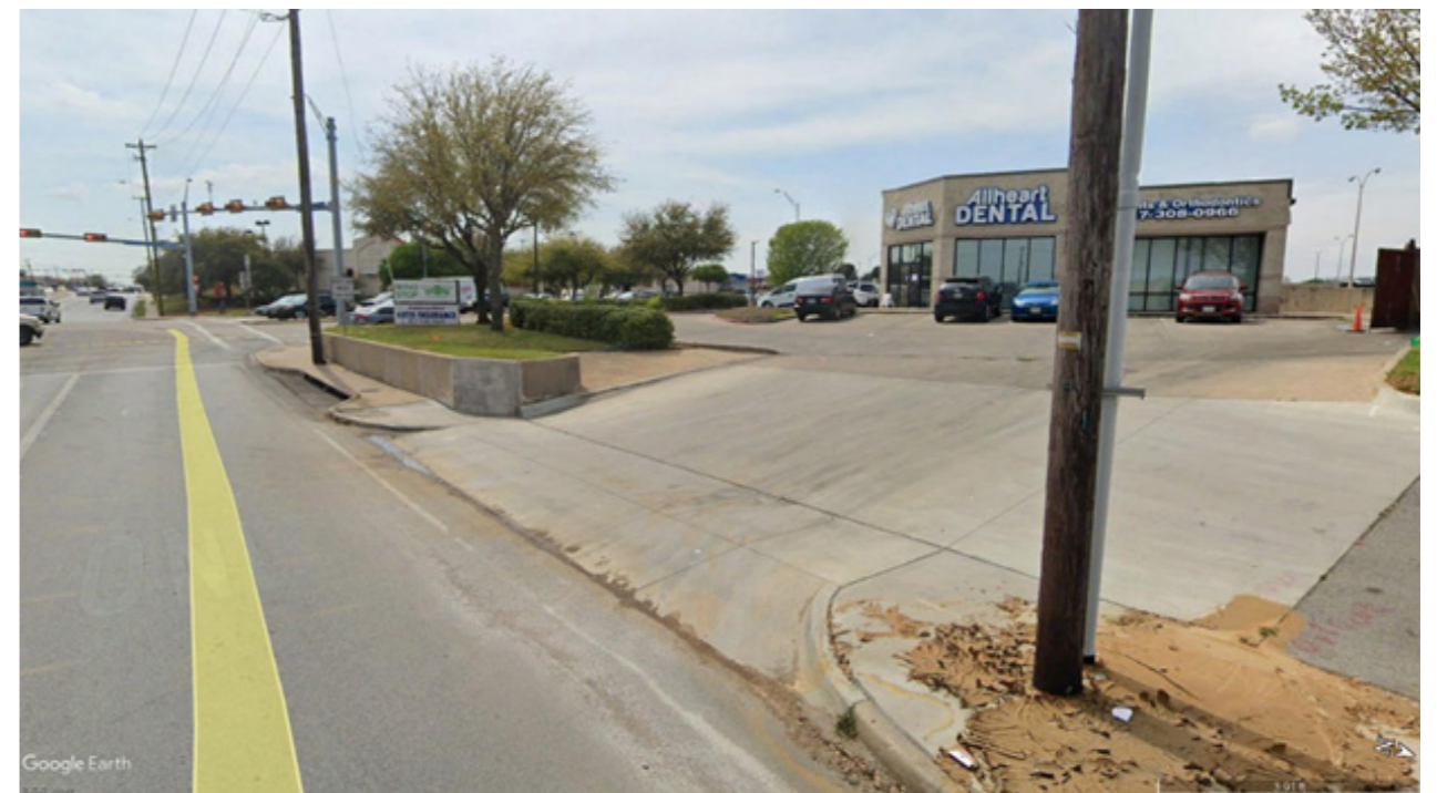
Figure 36: Sidewalk Near Cooper Street and Pioneer Parkway Source: Google Earth, AECOM, 2020
