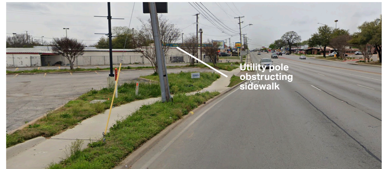
Figure 68: Examples of a Utility Pole in the Access Way near Cooper St and Arkansas Ln Source: Google Earth, 2020
